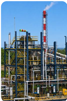
Solar DHF Plant
