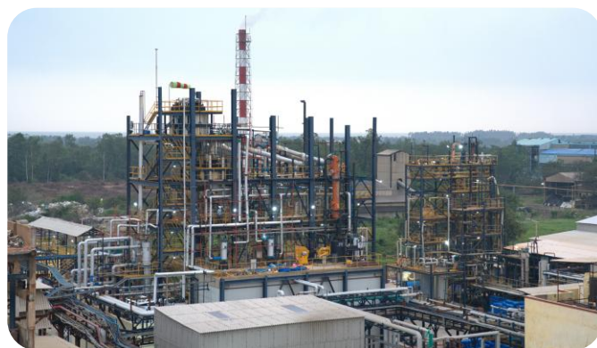
Solar DHF Plant
