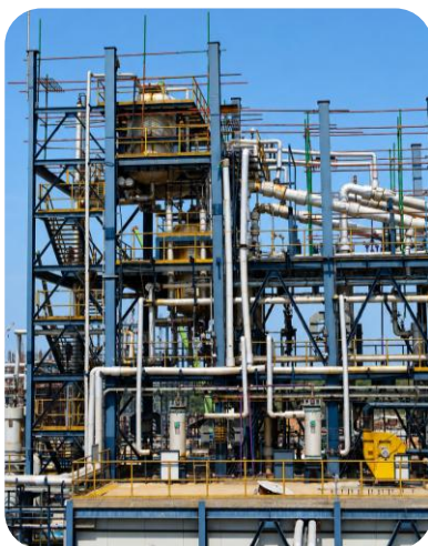
Solar DHF Plant
